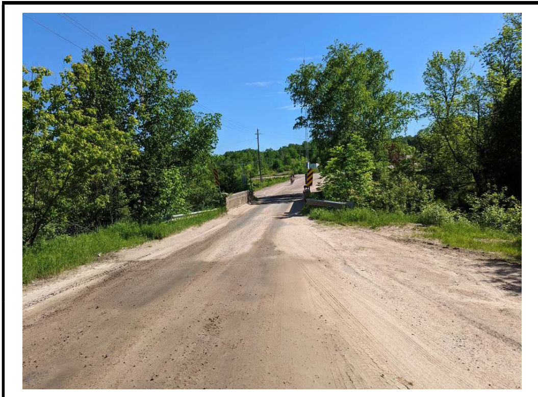
Photo 2 Structure from west approach
