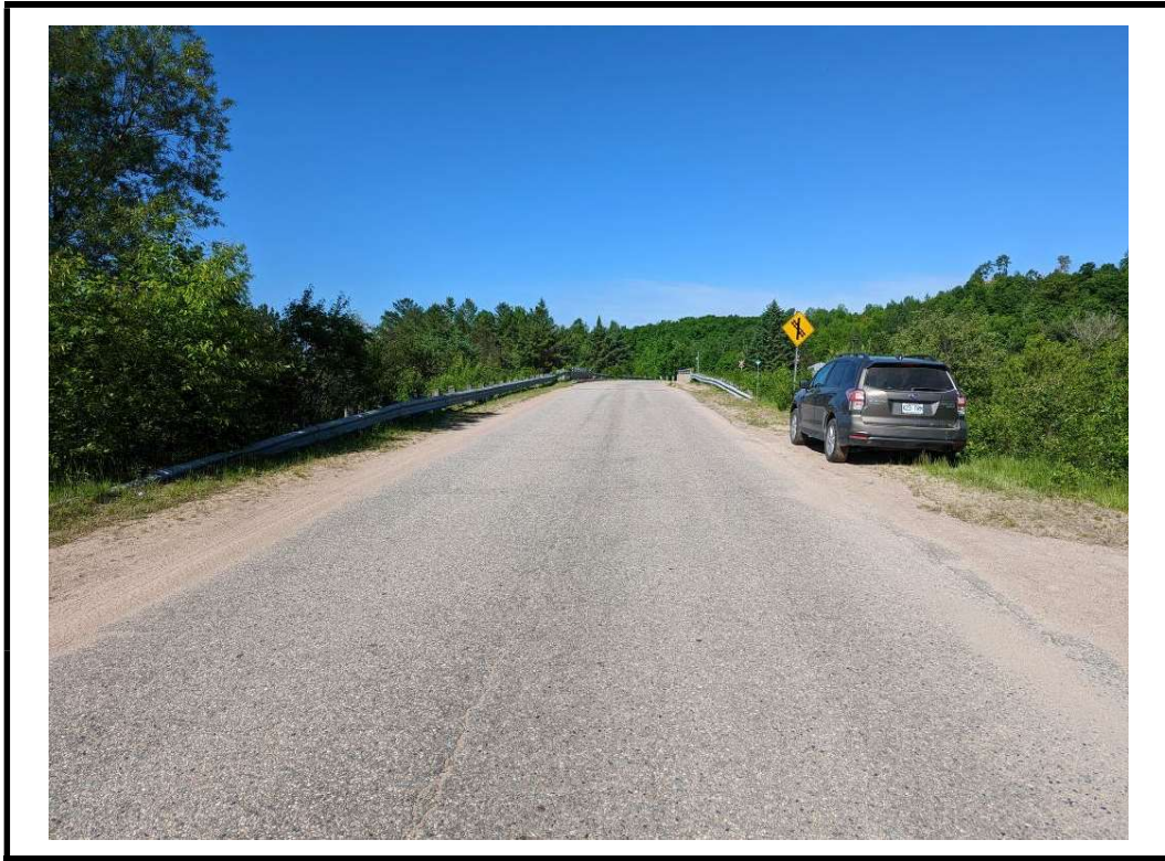
Photo 1 Structure from east approach
