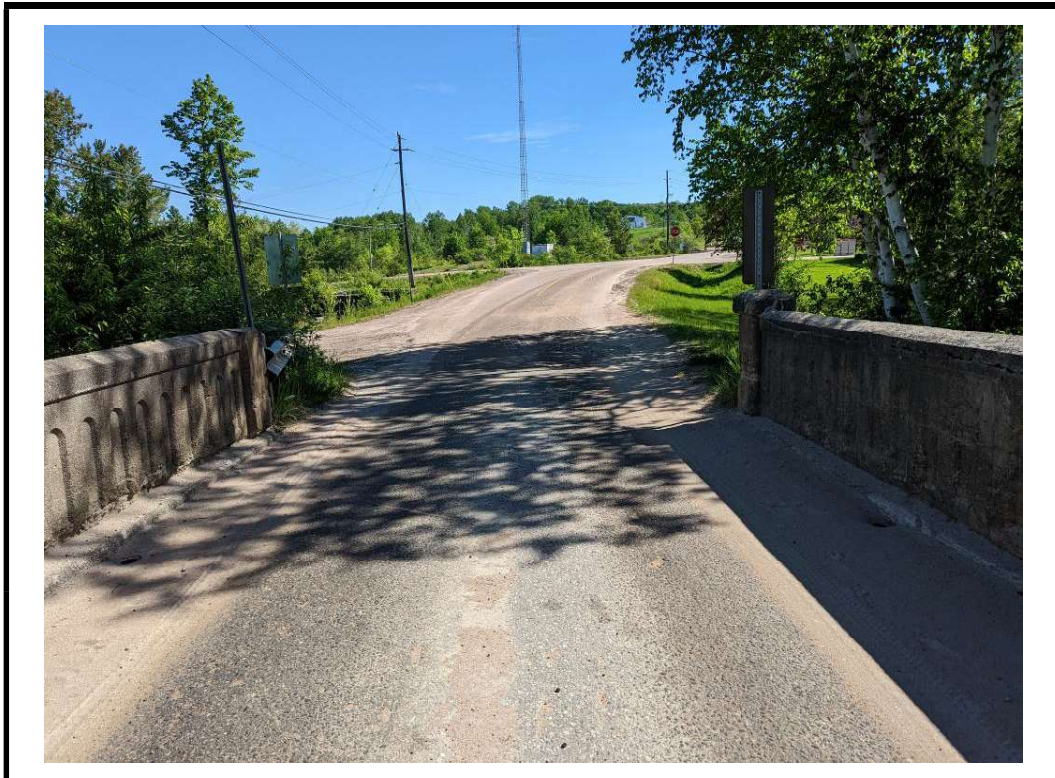
Photo 4 West approach from centre of structure
