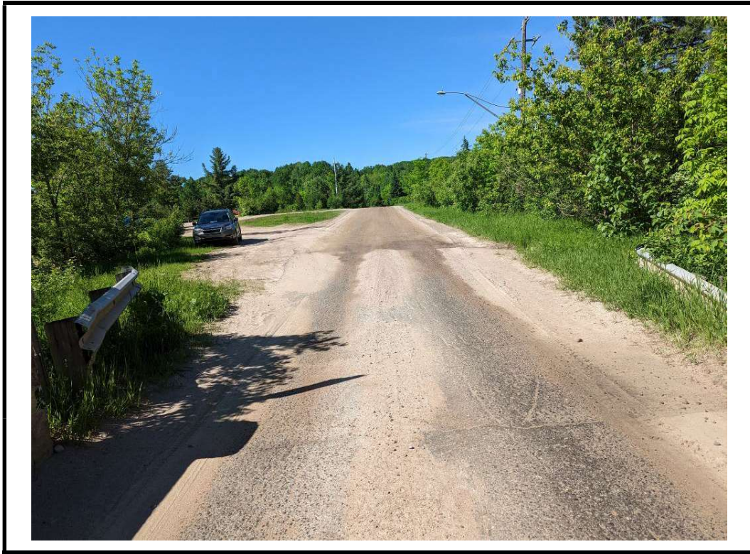
Photo 3 East approach from centre of structure
