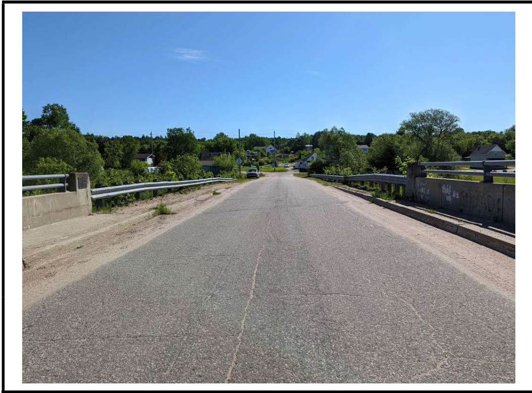
Photo 3 East approach from centre of structure
