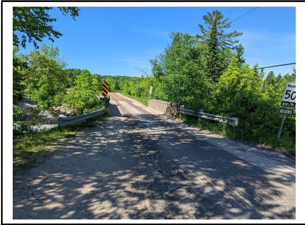
Photo 1 Structure from east approach
