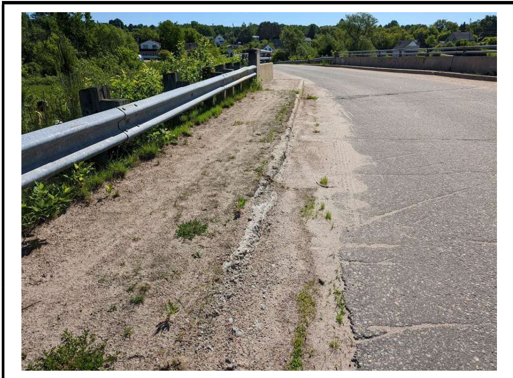
Photo 2 Structure from west approach
