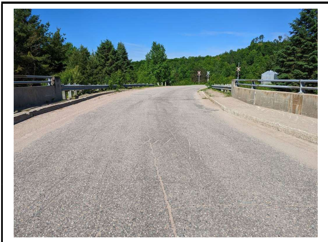
Photo 4 West approach from centre of structure
