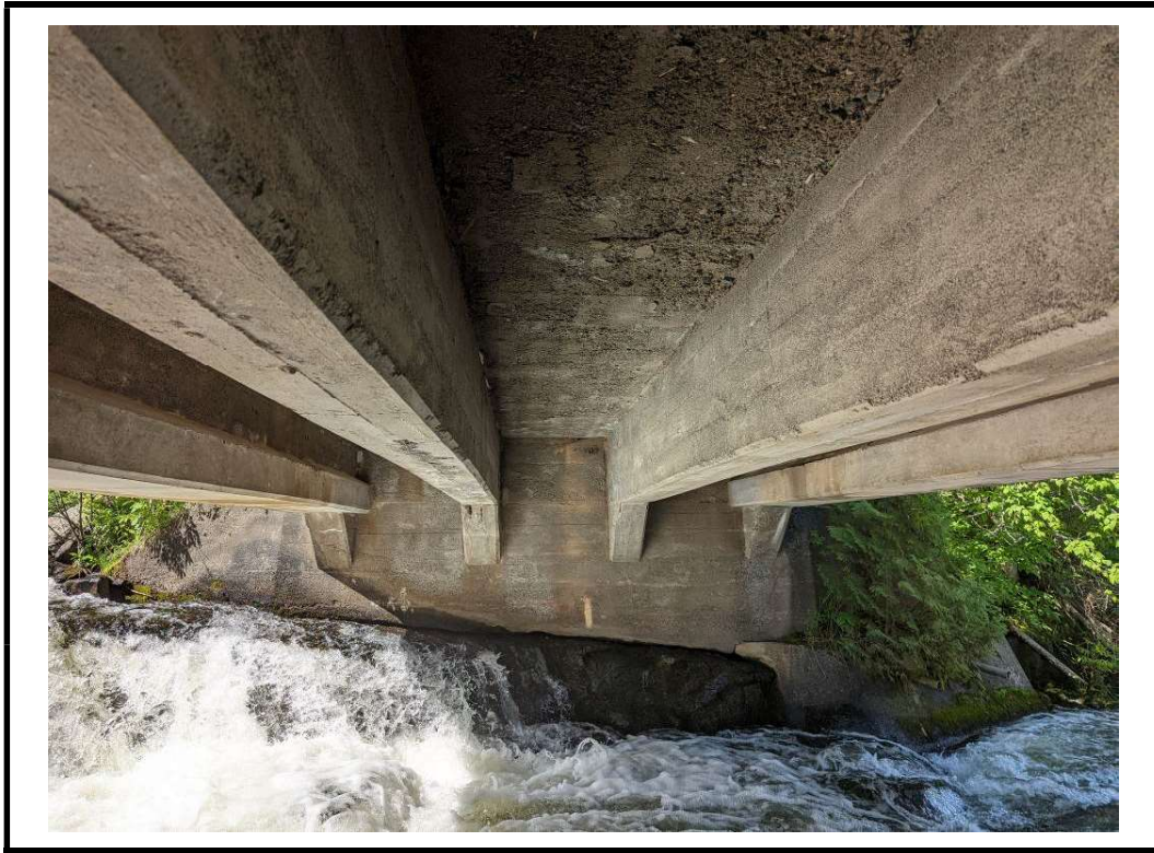
Photo 15 West underside of Structure
